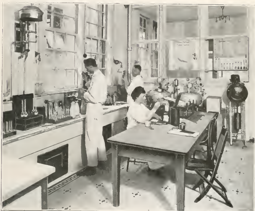
One of the laboratories where samples of milk are taken to be analyzed as to fat content, sediment, acidity, and bacterial count.
